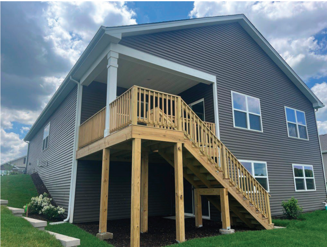
Photo 4: Looking South at Rear Deck and Rear Elevation
