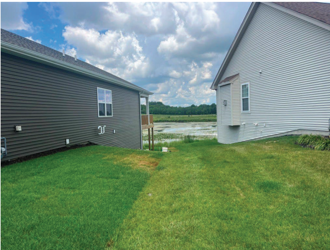
Photo 2: Looking Northwest Along Side Building Elevation
