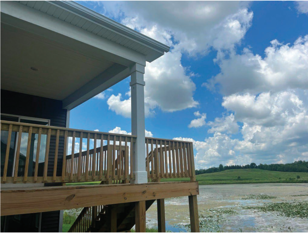
Photo 3: Looking Northwest at Rear Deck
